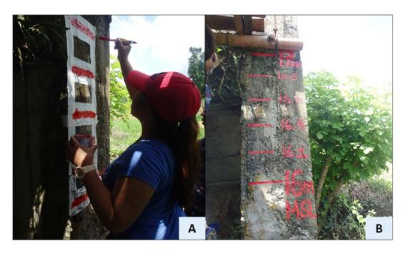
Figure 47. MSL water level markings at Hanging Bridge's Foot
