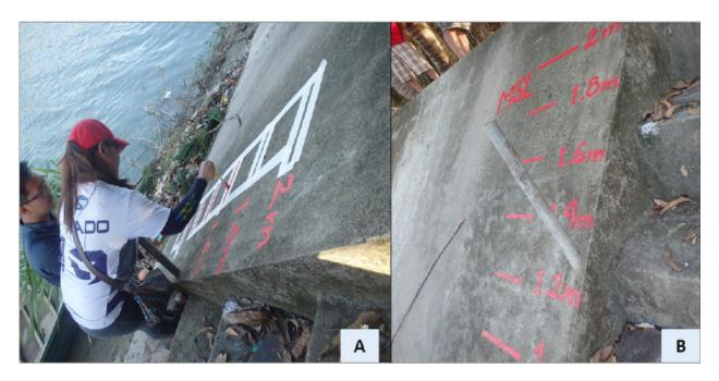
Figure 46. MSL water level markings at Labangan Bridge's Abutment
