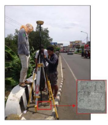
Figure 35. GNSS receiver occupation, Trimble® SPS 882 at ZN-44, Miputak Bridge, in Brgy. Miputak, Dipolog City, Zamboanga del Norte
