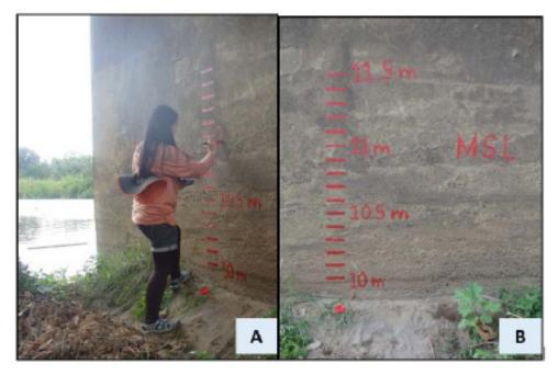
Figure 42. MSL water level markings in Polanco Bridge's Pier
