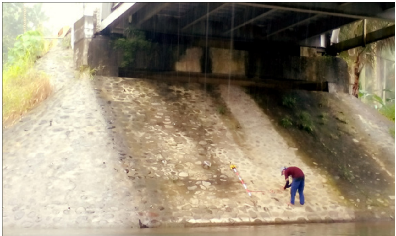
Figure 40. Water level marking on the abutment of Magsaysay Bridge
