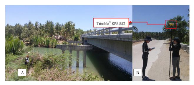
Figure 37. (A) Talisay Bridge facing upstream and (B) cross-section Survey using Trimble® SPS 882 in PPK survey technique
