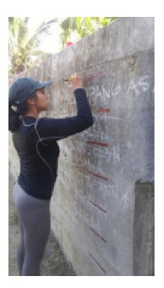
Figure 41. Water-Level Marking at Talisay Bridge
