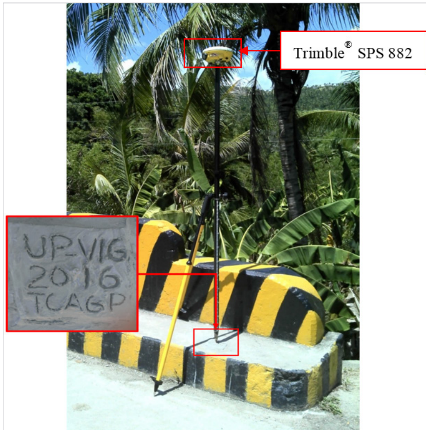
Figure 40. GNSS base set up, Trimble® SPS 882, at UP-VIG, located at the approach of Vigo Bridge in Brgy. Vigo Central, Municipality of San Francisco, Quezon.
