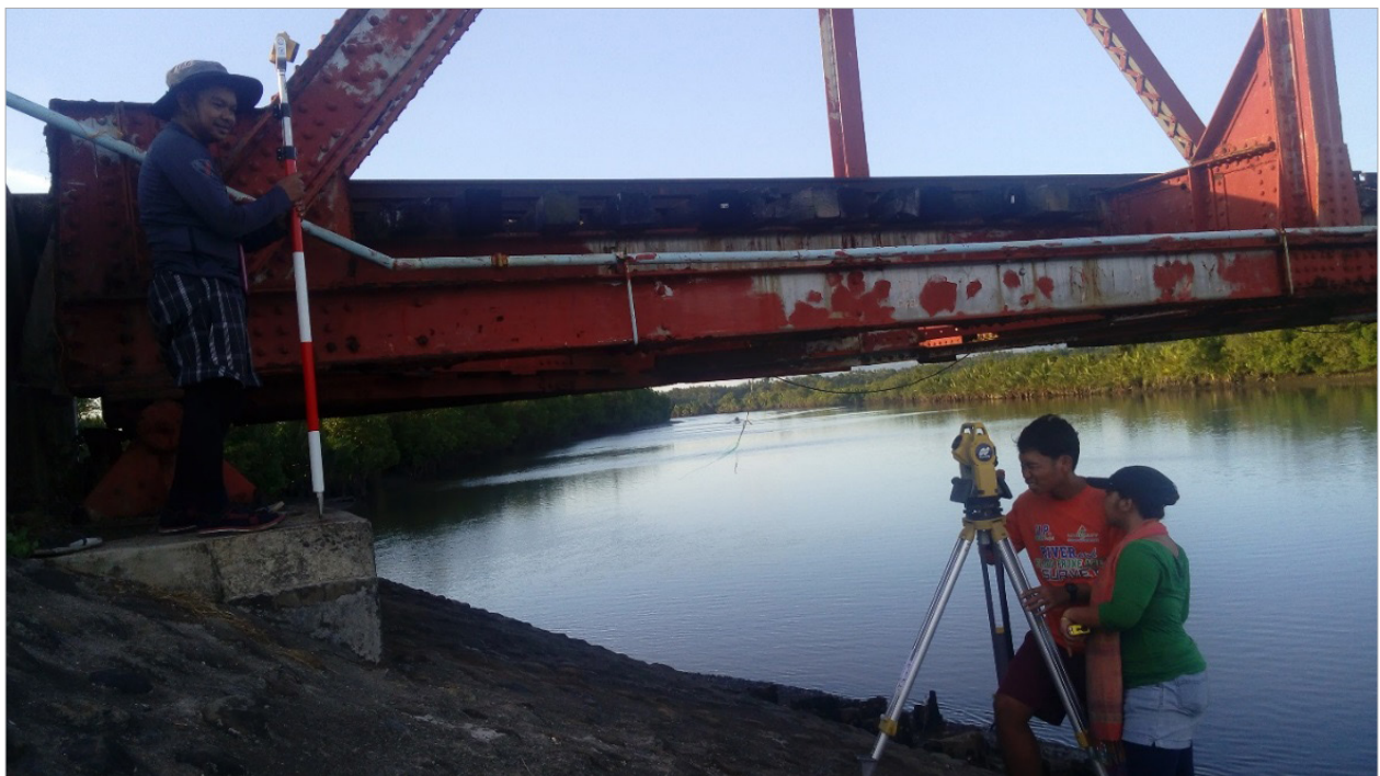
Figure 41. Cross-Section Survey for Vinas (also known as Cabibihan River) using Trimble® Total Station, in Open Traverse Method.
