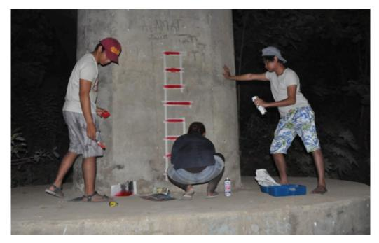
Figure 37. Water level marking at Kanguinsa Bridge
