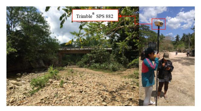
Figure 36. Kanguinsa Bridge and the actual cross-section survey using Trimble® SPS 882 in PPK survey technique
