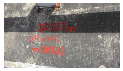
Figure 37. Water-level markings on Kilbay Bridge.
