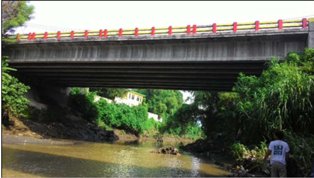
Figure 36. Imus Bridge facing upstream
