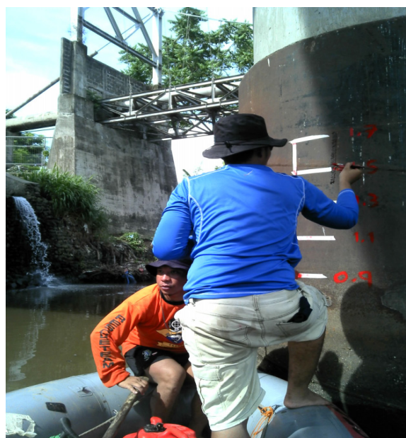
Figure 43. Marking of MSL-based elevation on the right side of a pier in Bridge of Promise
