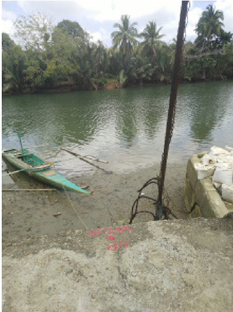
Figure 34. Water-Level Markings on the pavement in Anibawan Bridge
