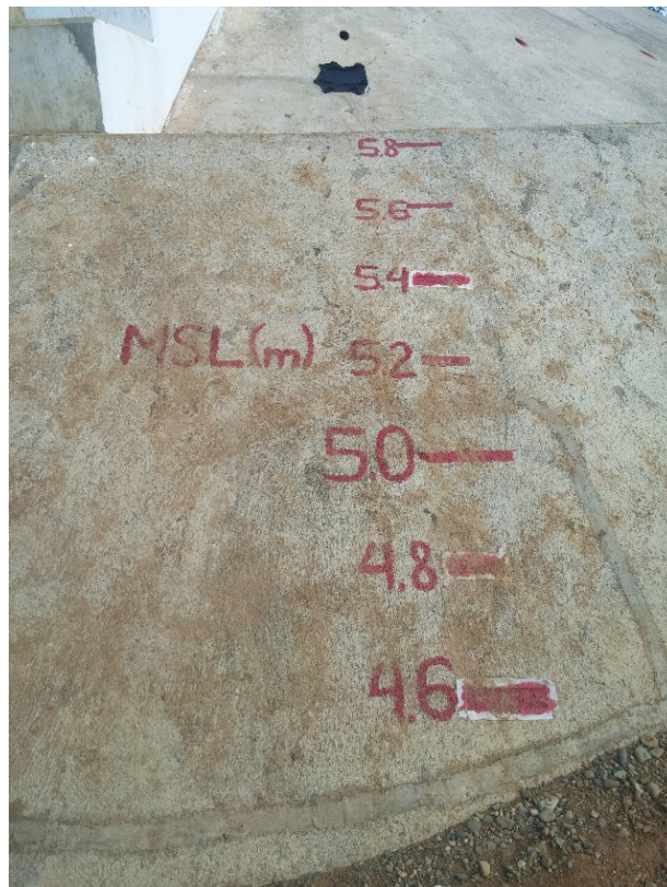
Figure 41. Water-level markings on New Pamplona Bridge
