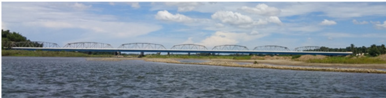
Figure 37. New Pamplona Bridge facing downstream
