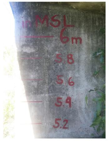
Figure 44. Water-level markings on the Linao Bridge
