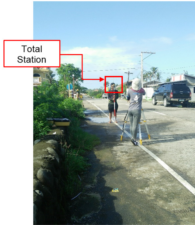
Figure 40. As-built survey of Casalugan Bridge
