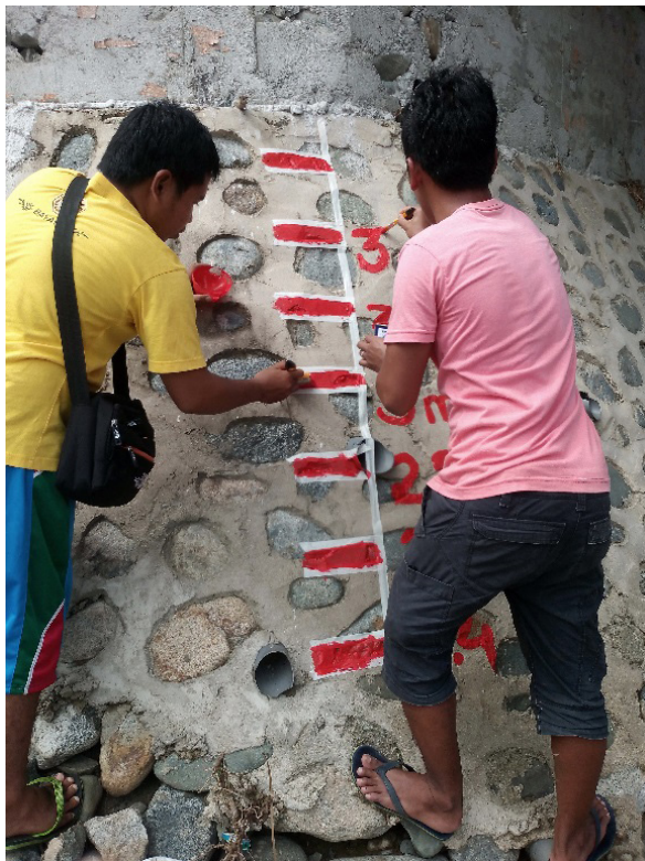
Figure 47. Water-level markings on Casiguran Bridge
