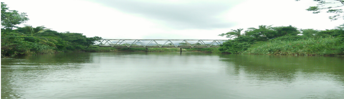
Figure 38. Casalugan Bridge facing upstream
