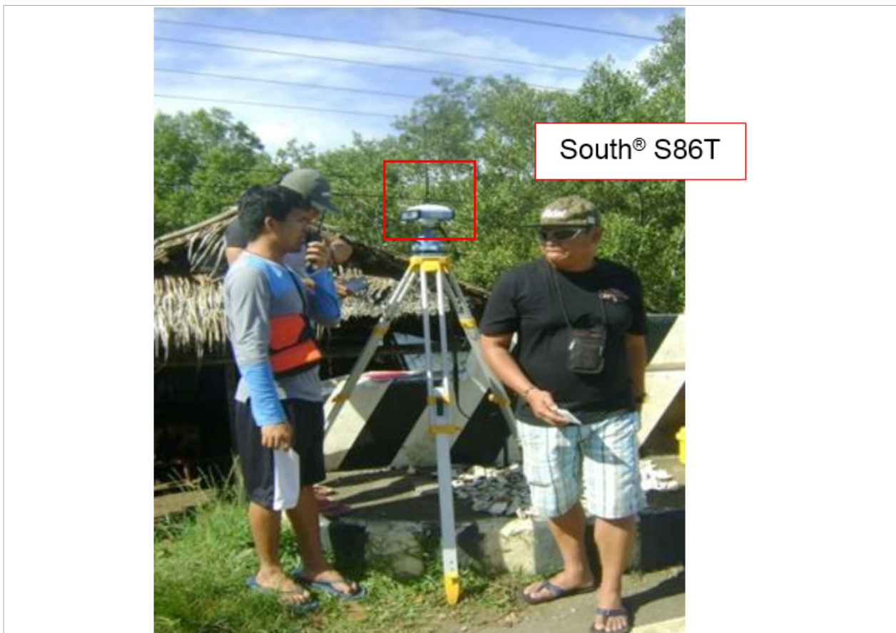
Figure 33. GNSS base receiver set-up, South® S86T, at SS-148 in Brgy. San Agustin Norte, Tandag City, Surigao del Sur
