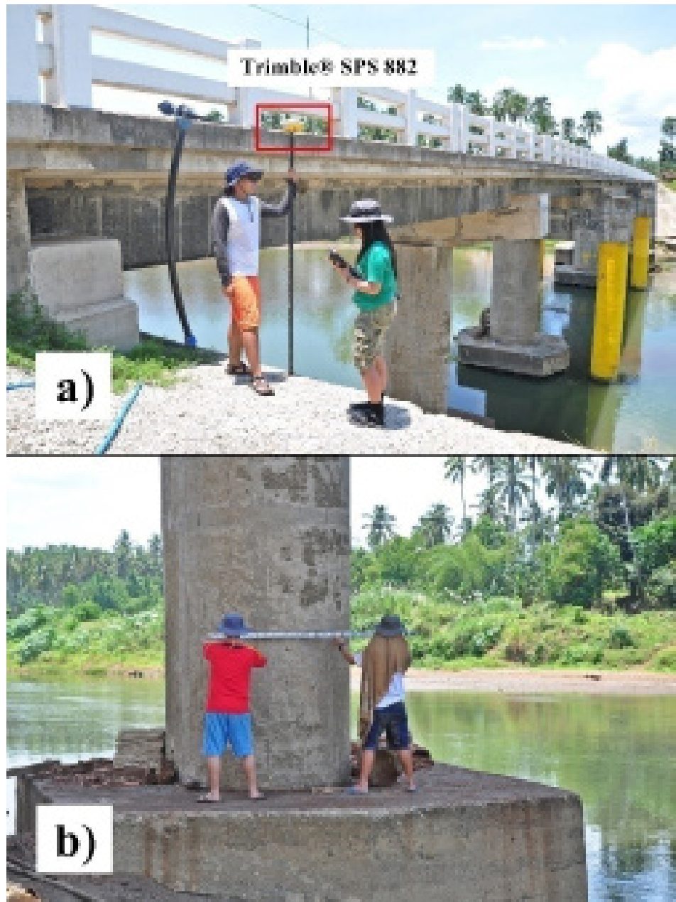
Figure 41. (a) As-built survey on the upper dike using Trimble® SPS 882 (b) measuring the width of one of the piers in Tago-San Miguel Bridge
