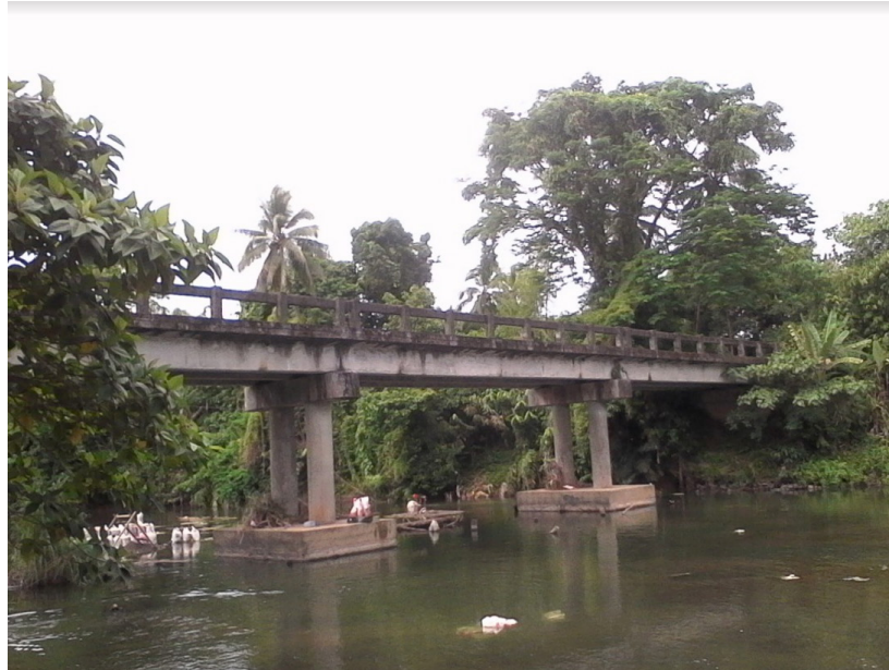
Figure 36. Kinabutan Bridge facing downstream
