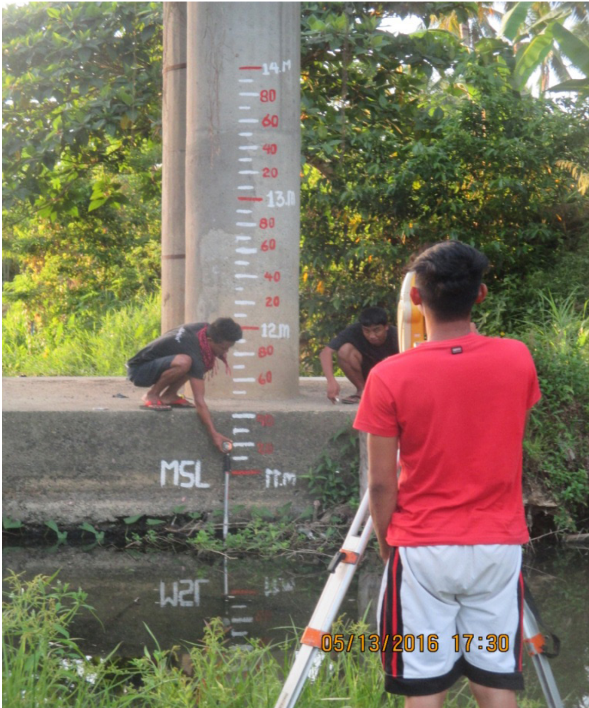
Figure 41. Water-level markings on Kinabutan Bridge.
