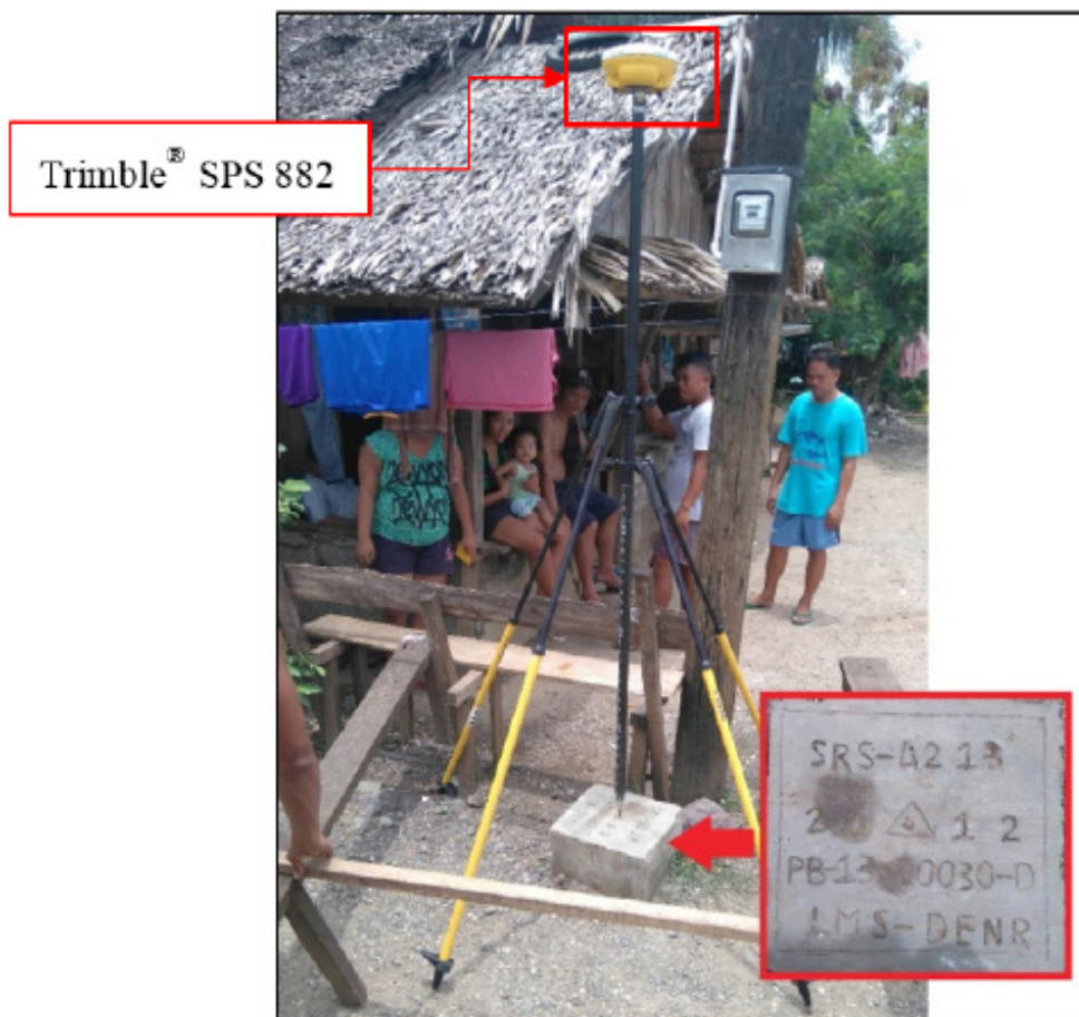
Figure 42. GNSS receiver set-up, Trimble® SPS 882, at BMSS-4213 located near the Burboanan Bridge in Barangay Burboanan, Bislig City, Surigao del Sur
