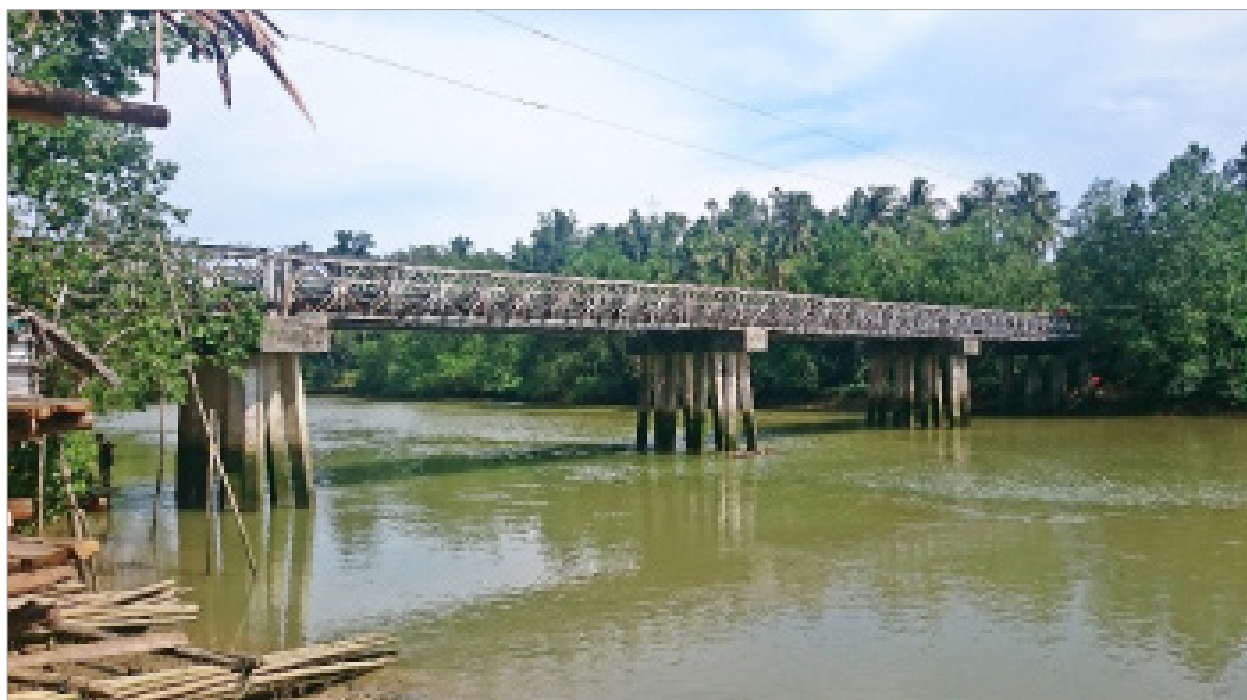
Figure 47. Hinatuan Bridge facing downstream
