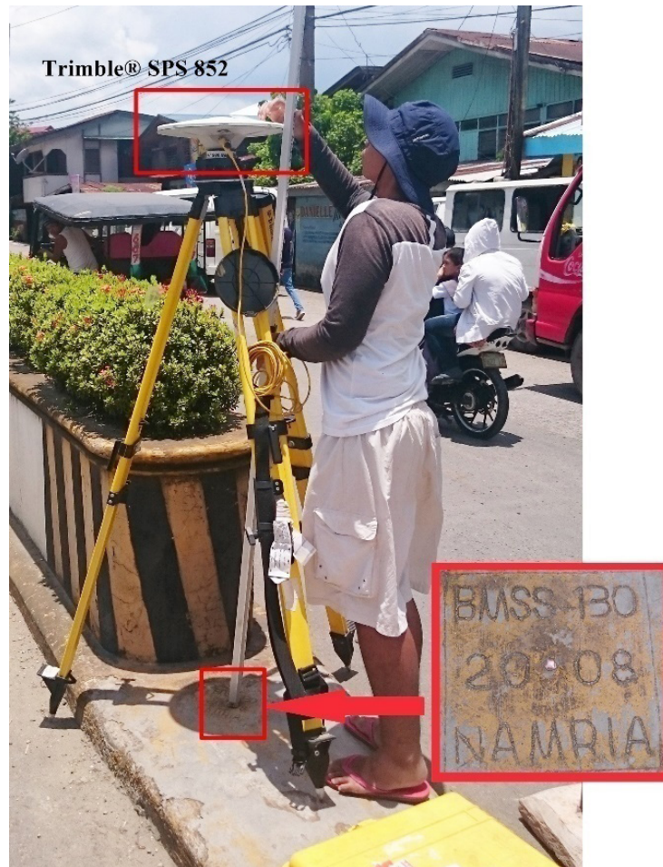
Figure 36. GNSS base set up, Trimble® SPS 852 at BMSS-130 located on one end of a concrete barrier along Surigao-Davao Coastal Road in Brgy. Mangagoy, Bislig City, Surigao del Sur
