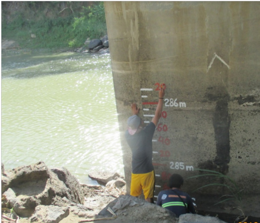
Figure 44. Water-level markings on Valencia Bridge
