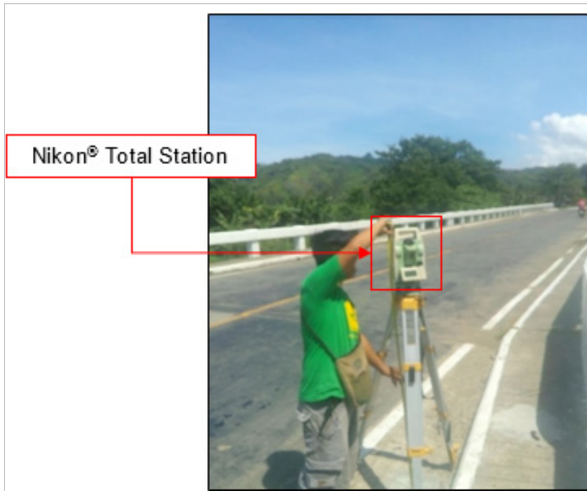
Figure 40. As-built survey of Valencia Bridge
