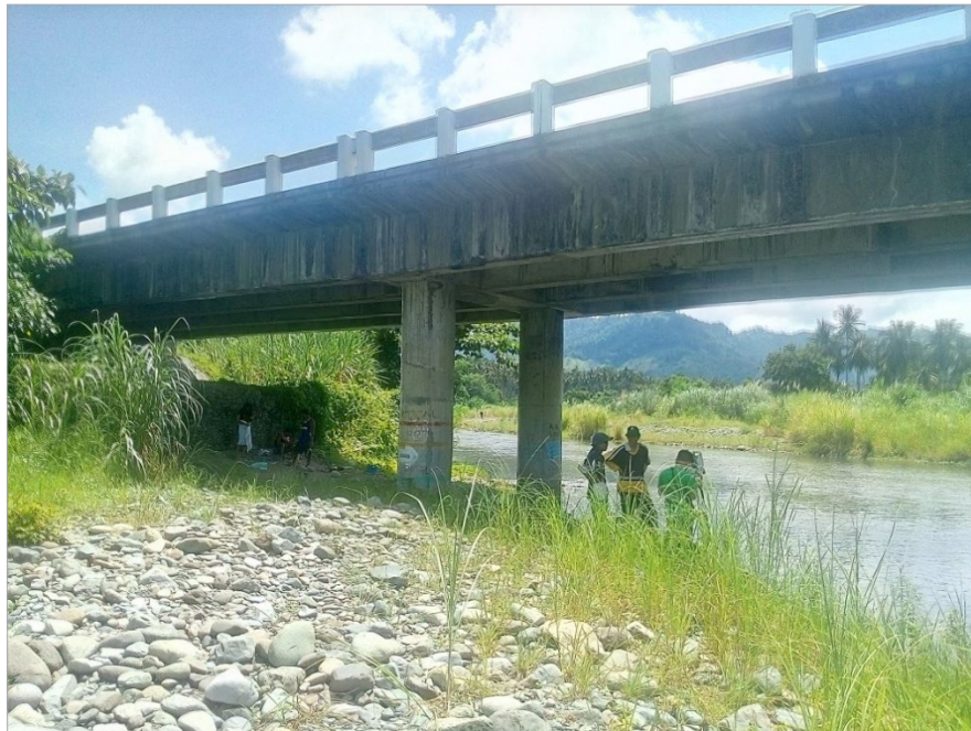
Figure 39. Upstream side of Valencia Bridge
