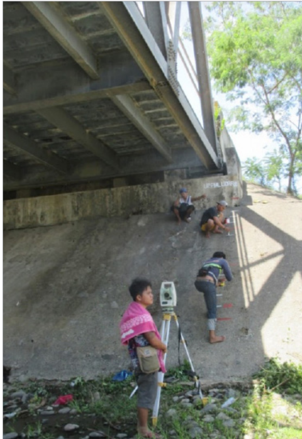
Figure 44. Sawaga Bridge facing upstream
