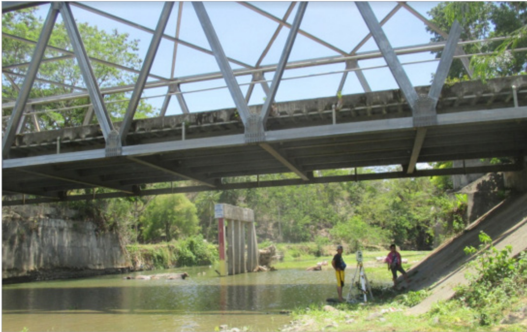
Figure 39. Sawaga Bridge facing upstream
