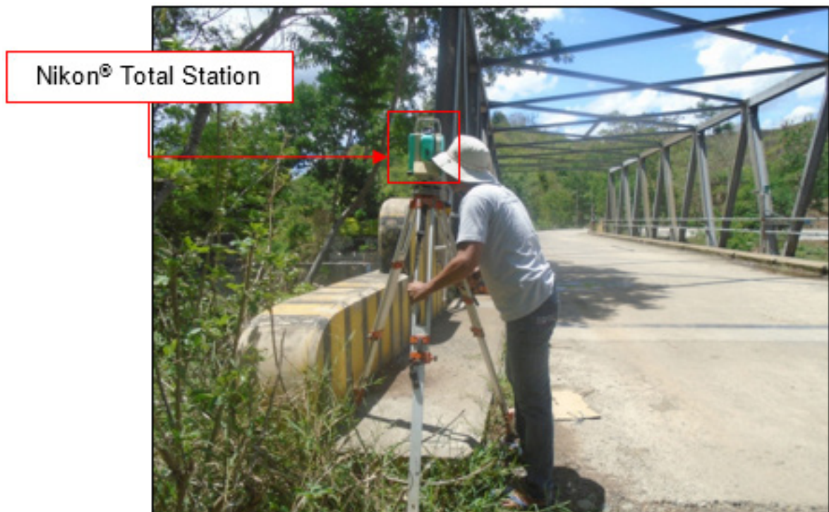
Figure 40. As-built survey of Sawaga Bridge
