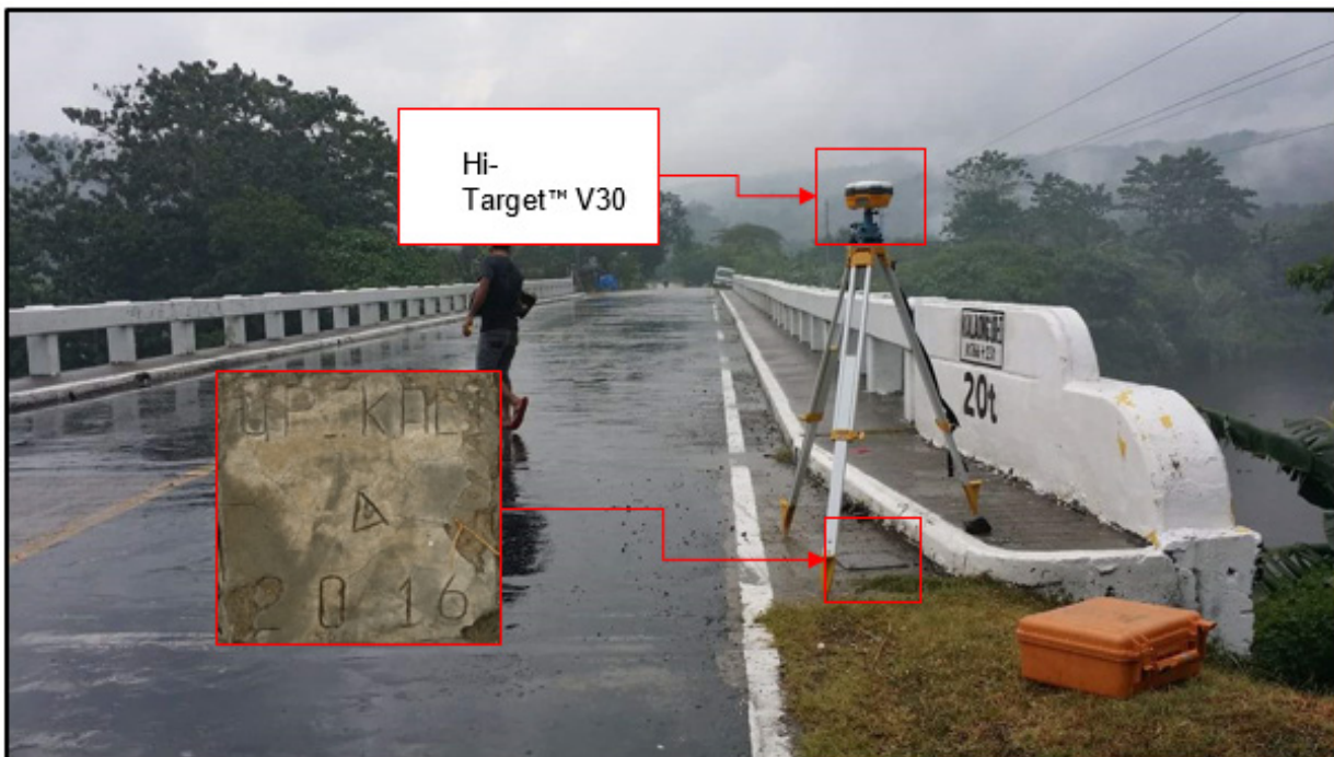
Figure 37. GNSS receiver set-up, Hi-Target™ V30, at UP_KAL-1, an established control point, located beside the approach of the Kalaong Bridge in Barangay Kalaong, Maitum, Sarangani.
