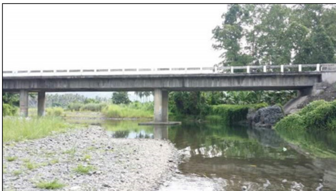
Figure 39. The Kalaong Bridge facing upstream.
