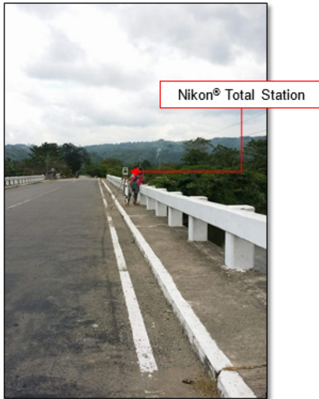
Figure 40. Bridge as-built survey of the Kalaong Bridge.
