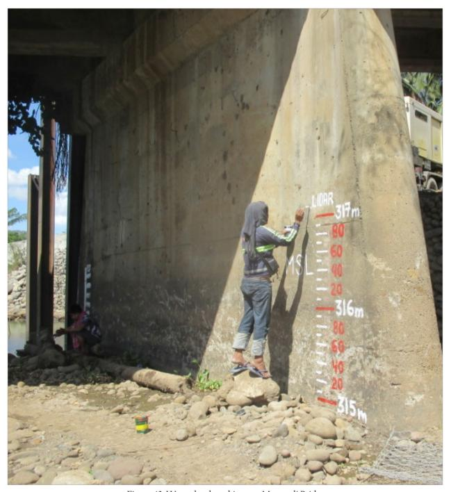
Figure 43. Water-level markings on Manupali Bridge
