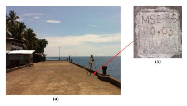
Figure 6. GPS set-up over MSE-36 within Medina municipal port(a) and NAMRIA reference point MSE-32 (b) as recovered by the field team
