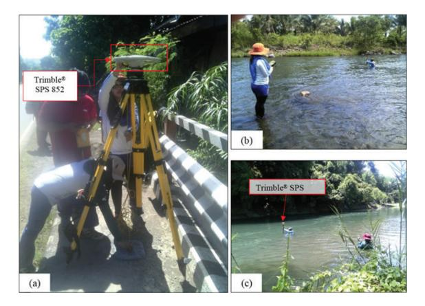
Figure 39. The bathymetric survey team preparation for the conduct of the bathymetric survey: (a) GNSS base station setup over CAB-1 in Cabulig Bridge, (b) gathering of bathymetry data downstream with respect to Cabulig Bridge, and (c) gathering of bathymetry data in the upstream
