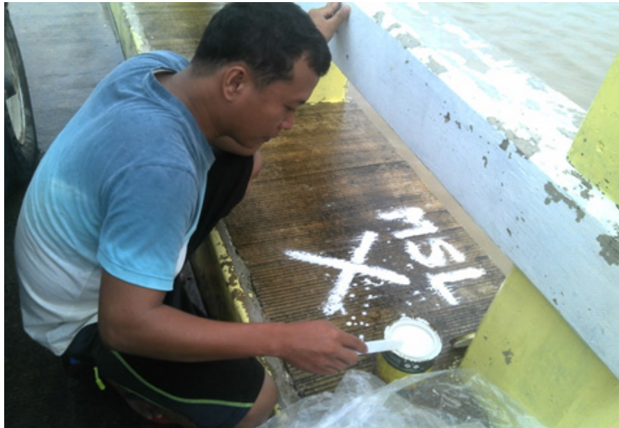
Figure 39. Water-level markings on the Umiray Bridge
