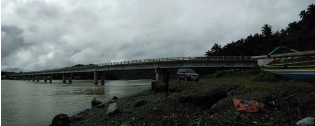
Figure 34. The Umiray Bridge facing downstream.
