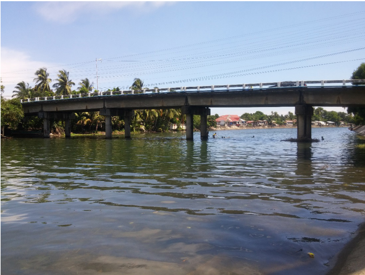
Figure 35. Morong Bridge facing downstream
