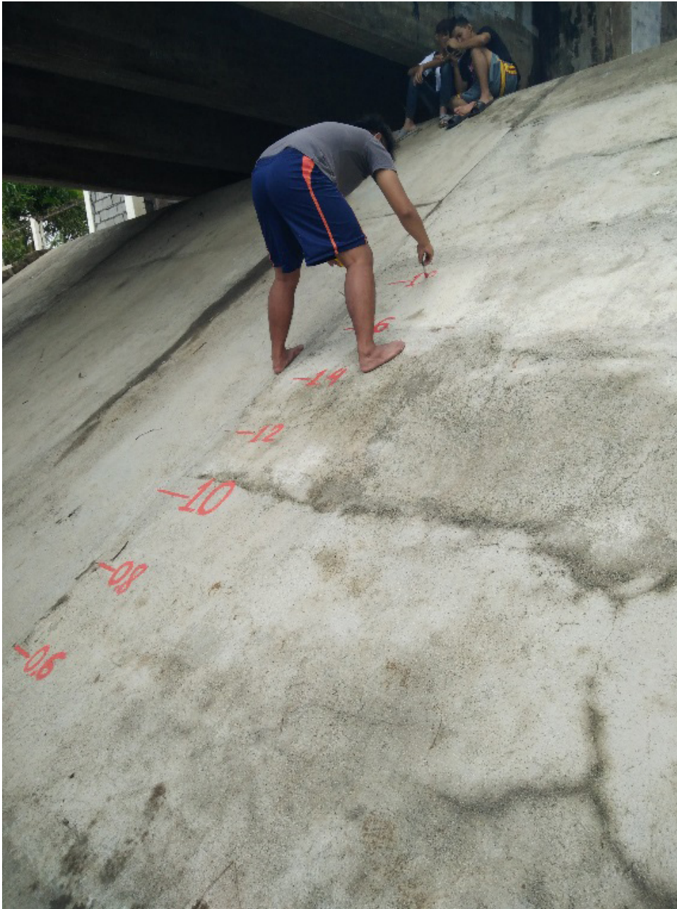
Figure 39. Water-level markings on Morong Bridge
