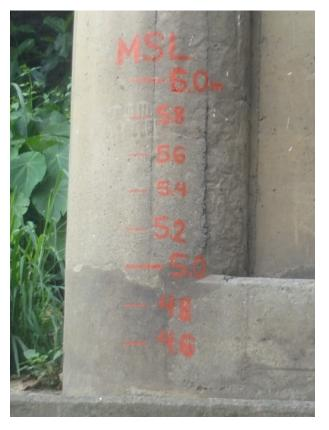
Figure 41. Water-level markings on Talisay Bridge
