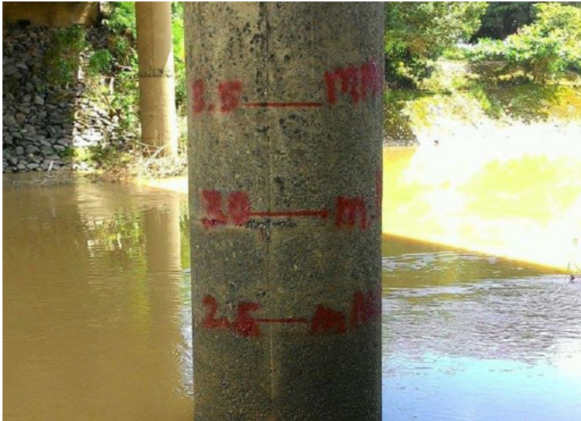
Figure 41. Water level marking on the pier of Gayaga Bridge
