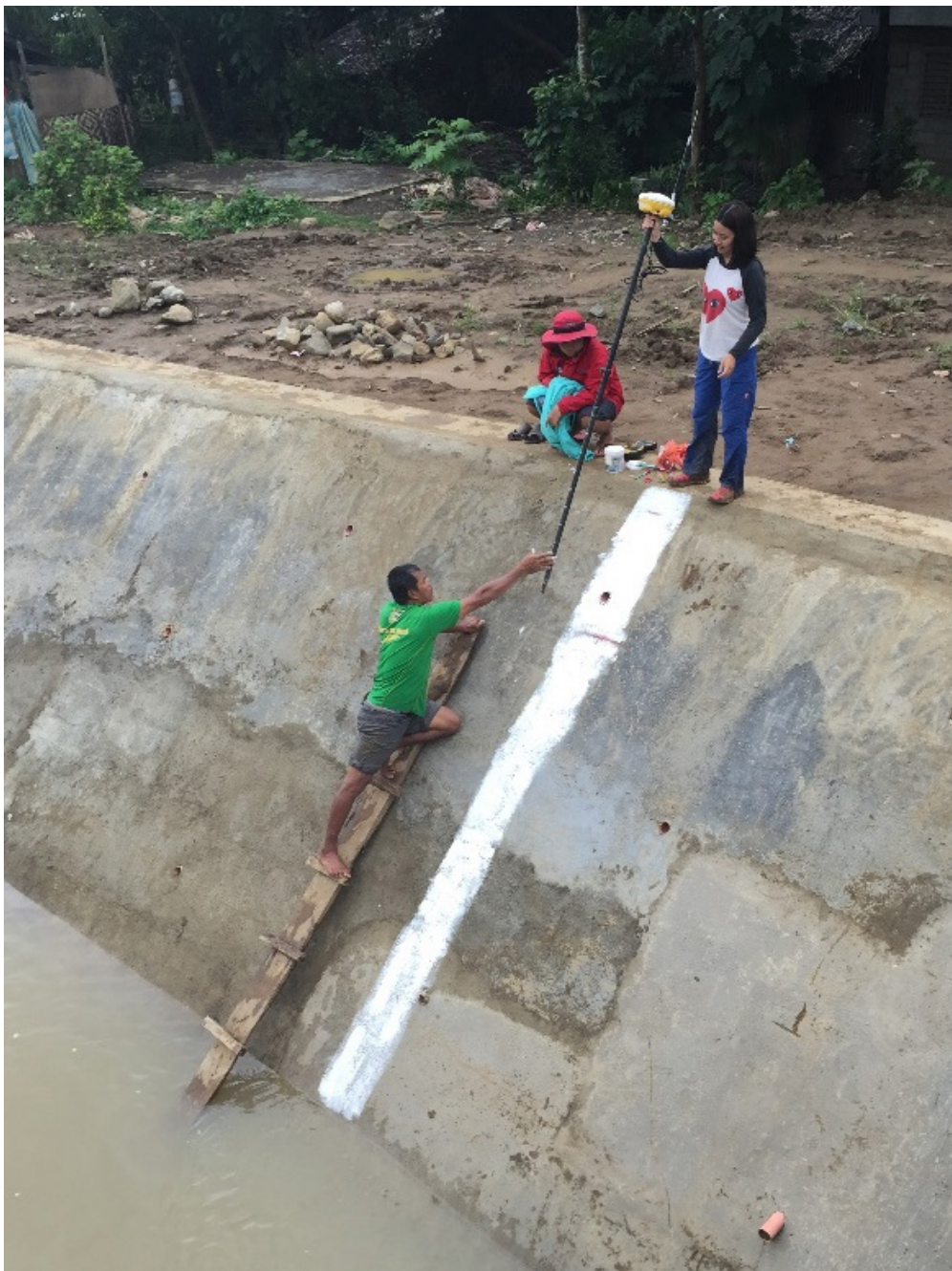
Figure 43. Water-level marking for Tupilac River
