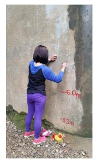
Figure 46. Water-level marking at Tigbao Bridge's Footing
