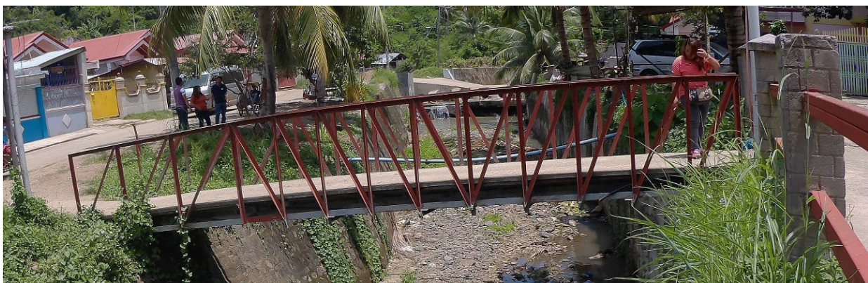
Figure 37. Townsville Bridge facing upstream
