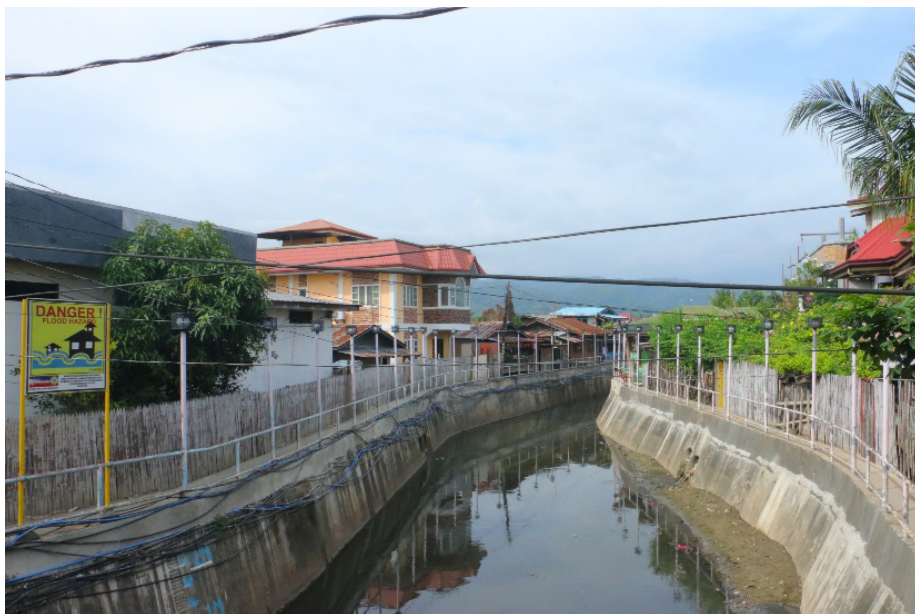
Figure 1. Concrete banks of San Jose River
