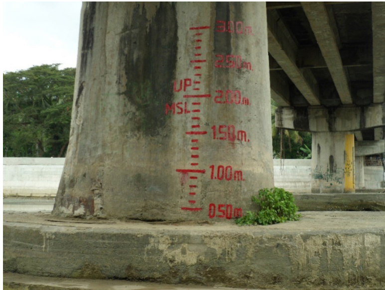
Figure 40. Water level marking at Salug Bridge
