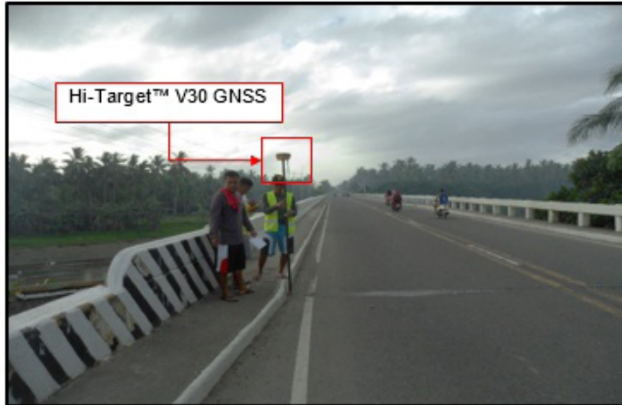
Figure 36. As-built survey of Salug Bridge
