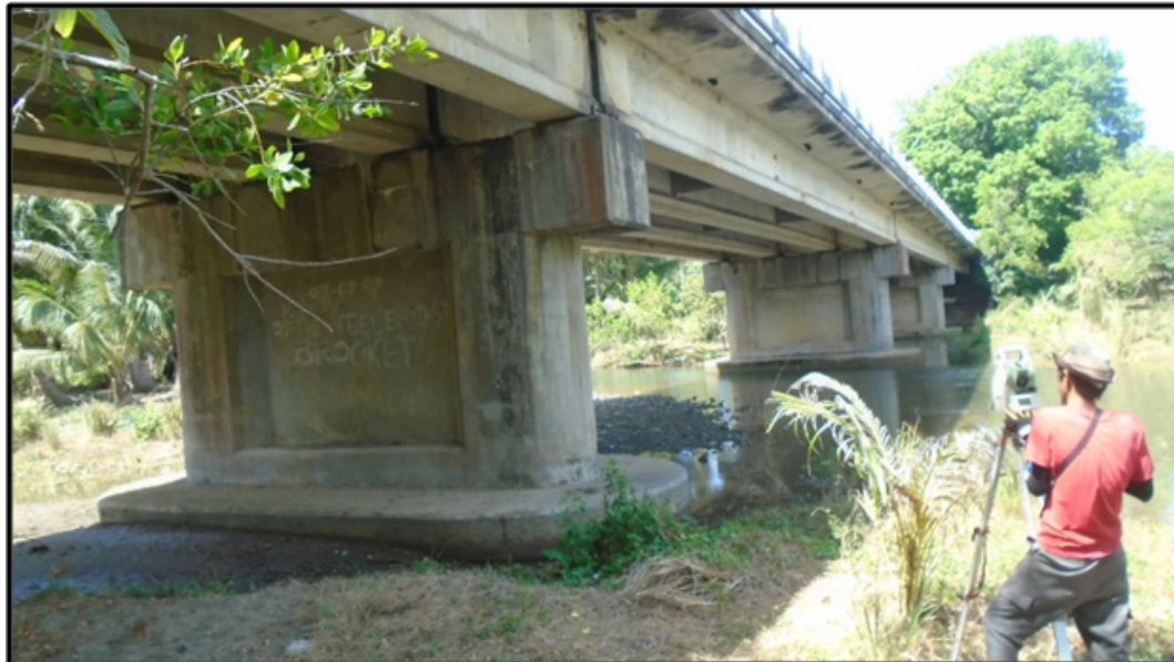
Figure 37. Figure C-9 Polandok Bridge facing upstream
