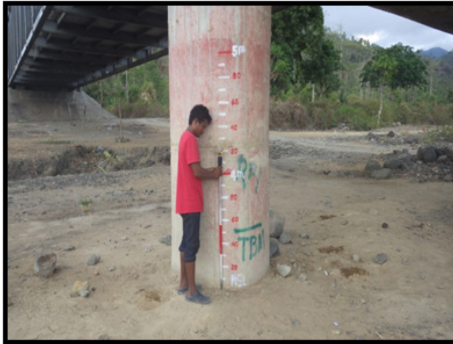
Figure 41. Water-level markings on Limpapa Bridge.
