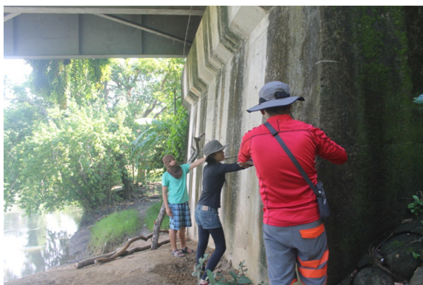
Figure 41. Water level marking on Ilog Bridge, Brgy. Gura, Donsol, Sorsogon.
