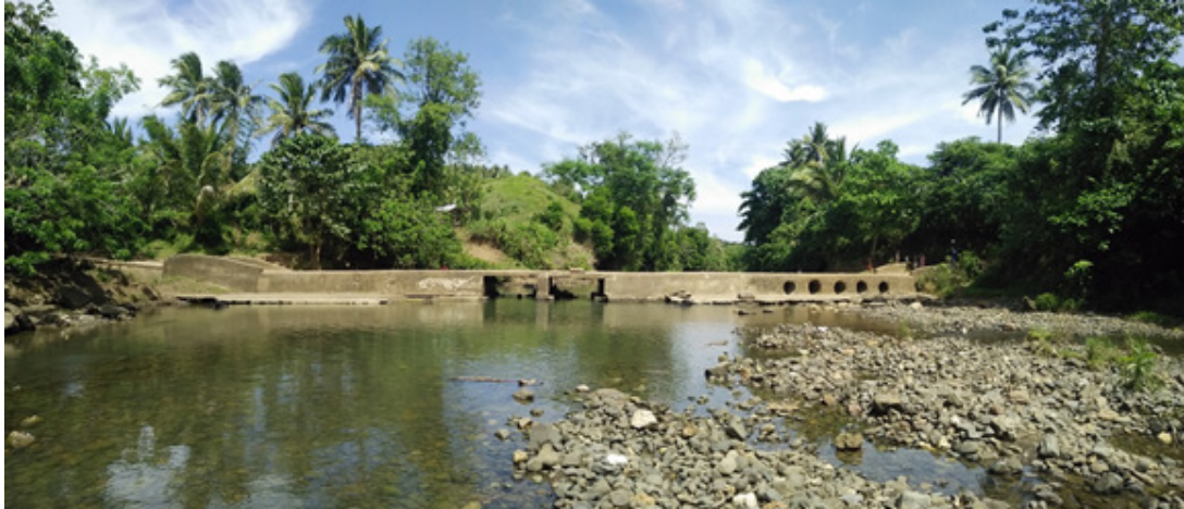
Figure 41. Malbag Culvert facing upstream
