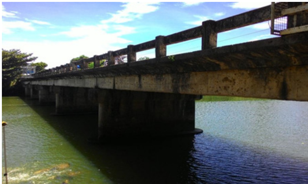
Figure 36. Mocong bridge facing downstream
