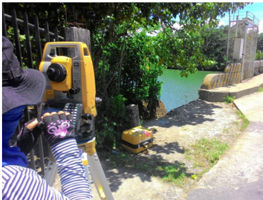
Figure 37. Mocong bridge as-built survey
